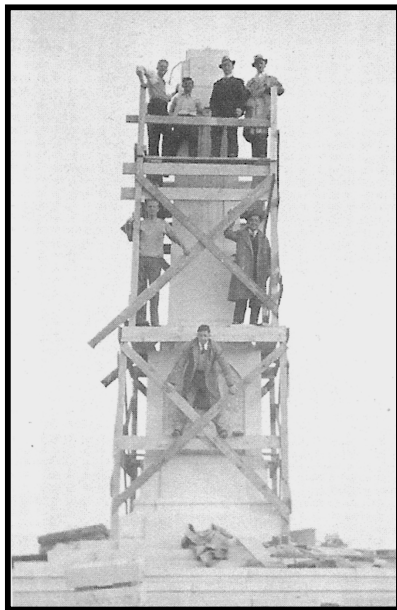
Scaffolding around the obelisk of the Monument
